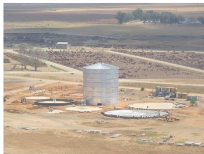
Construction of Reactor Tanks
